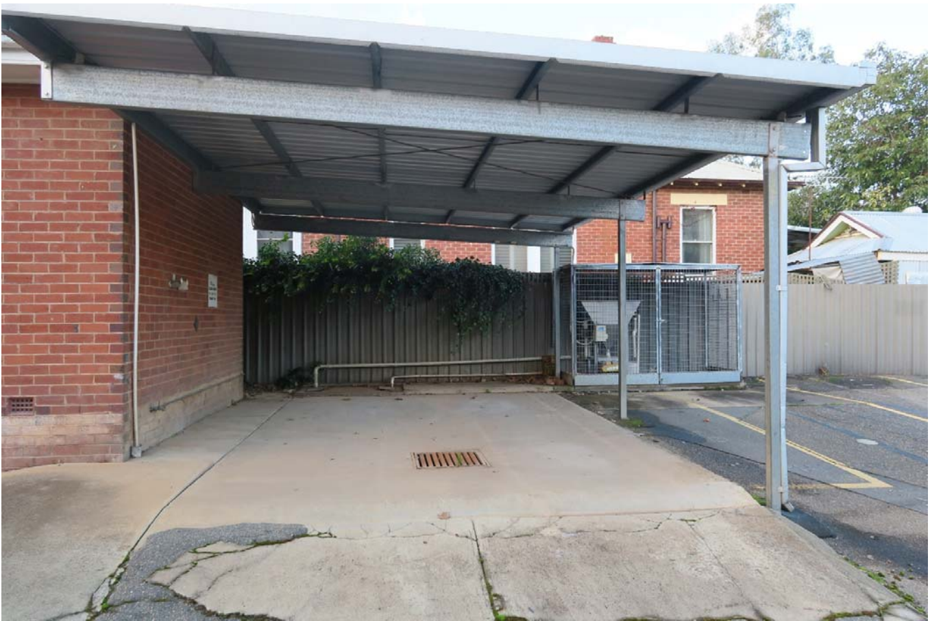
Covered wash bay at the southern end of the Laboratory building (north east corner of the site). The wash appears to drain to a waste water treatment system visible against the colourbond fence to the right (south) of the wash bay.
