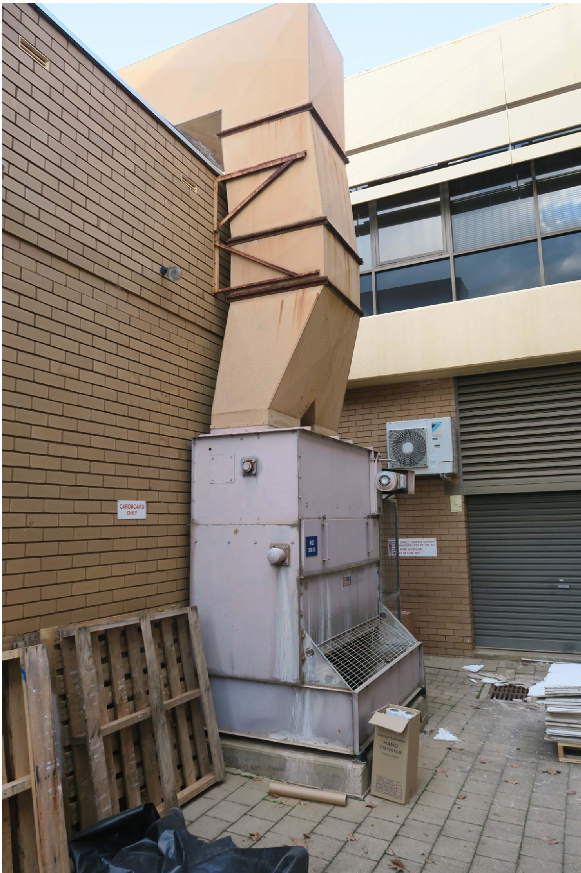
Extractor fan on the laboratory building.
