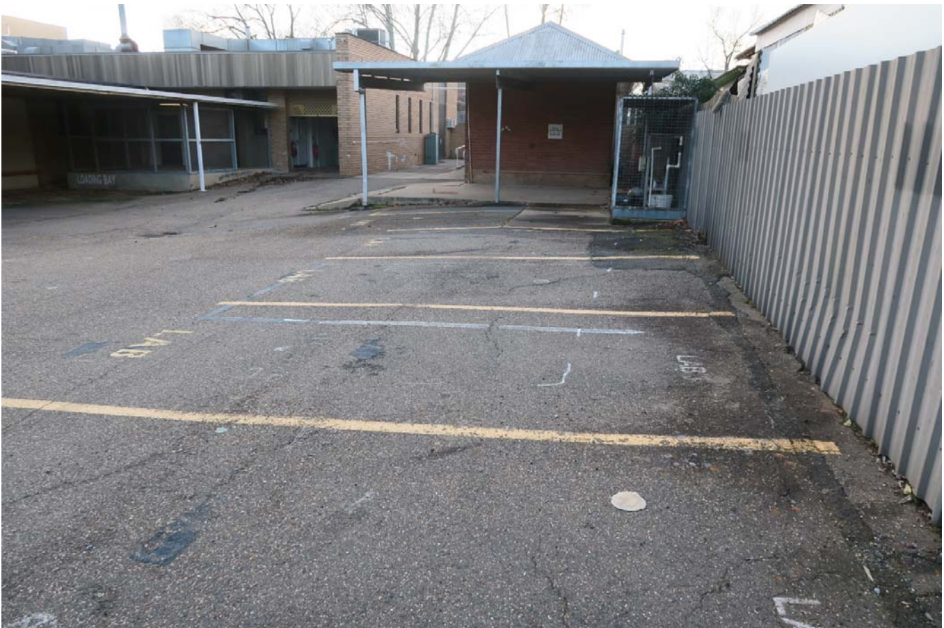
Suspected UST location adjacent to the eastern boundary. Previous borehole locations were evident in the asphalt surface of the car parking areas.
