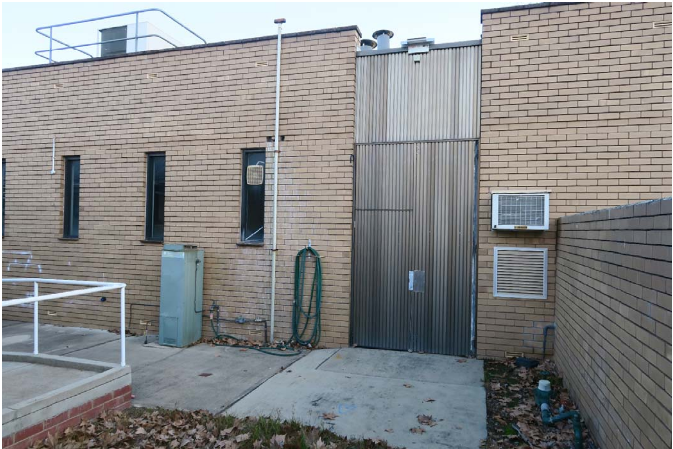
The north east corner of the Laboratory building showing what was thought to be a former plant room. A vent pipe was mounted to the building and is typical of a vent for a diesel storage UST. Documents identified in the SafeWork indicate a SUST was removed from this area in 1995. It is likely that the UST was removed and the vent left in place.
